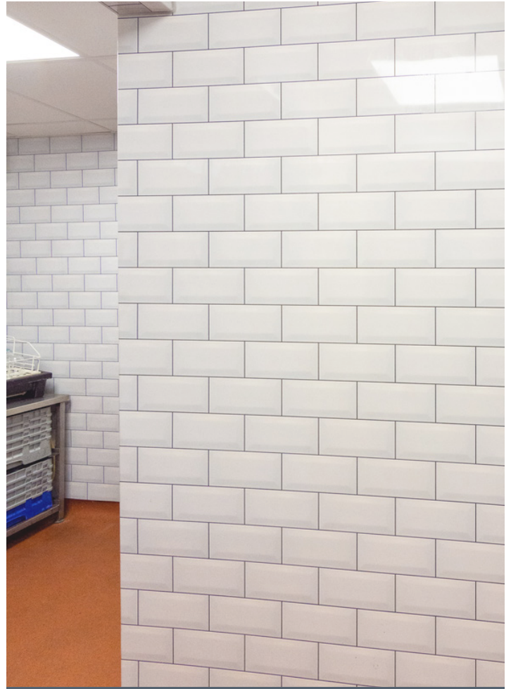
METRO WINSLOW INSTALLATION
